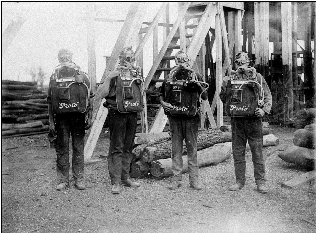
Figure 6: Fire investigation team wearing 'Proto' breathing apparatus at the C.S.A. mine in 1920. L to R: Fred Rue (miner) A.J. Julius (Mine Manager), Gwyder Whalen (surveyor), Bob Pivetta (underground foreman).
