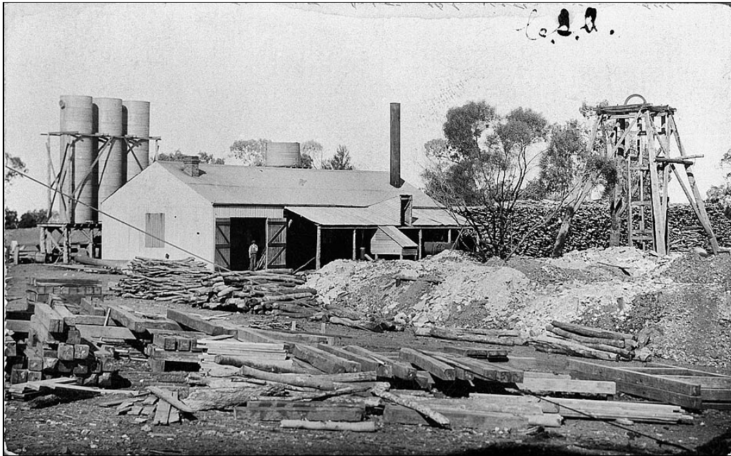
Figure 3: View looking southeast of the discovery shaft (original main shaft) and plant at the C.S.A. mine ca. 1908. Note the steam condensers at rear of engine house and timber for the underground workings.
